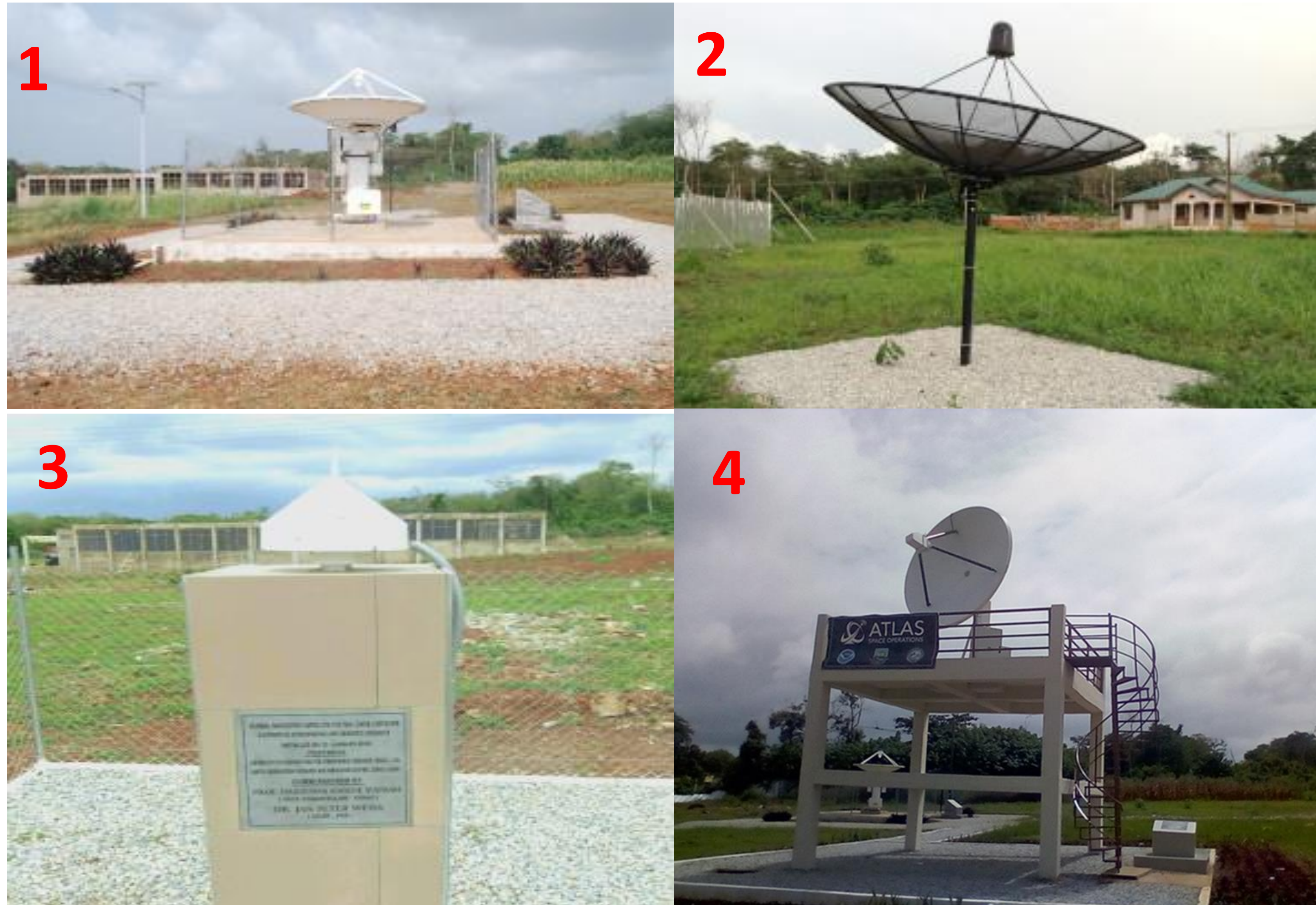
Fig 1: Earth Observing System – Direct Broadcast Ground Receiving Station (1), GEONETCast Reception Station (2), GNSS Referencing Station(3), COSMIC-2 Ground Station (4)
